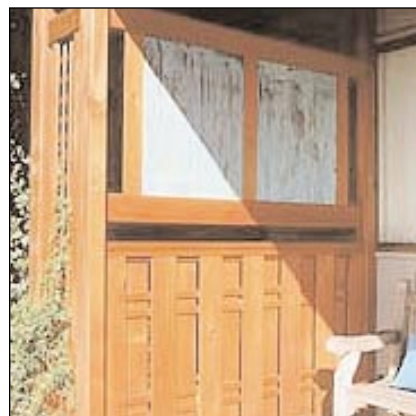
This redwood screen was constructed to hide a garden tool area at one end of a patio, and features custom latticework and copper inserts that have been chemically aged to a rich turquoise patina.
