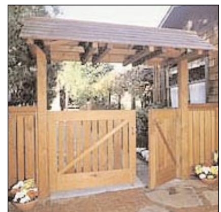
Rooftop-style canopy over a Craftsman fence shelters the entrance beneath it. Shingles on the canopy echo the design of the home. Posts are 6x6's and support the 4x4's of the canopy.
