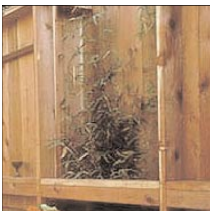
The extra deep window box acts like a greenhouse window, brightening the classic board-and-board fence. It also provides a showcase area for plants and flowers.
